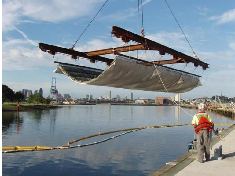
Figure 19 Tensar® Mat Being Installed.
