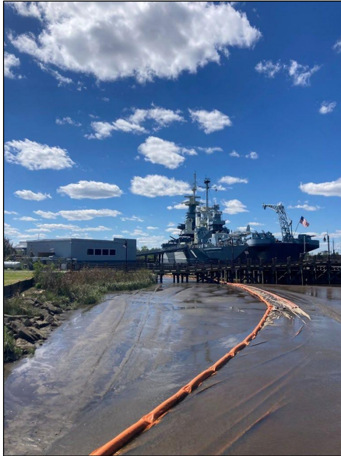
Appendix A-1. Silt boom near kayak launch.
