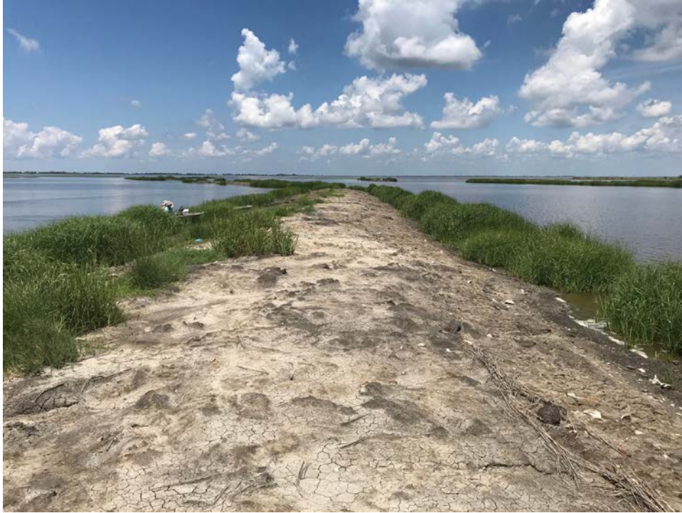
Figure 30. Terrace at the Pointe aux Chene site illustrating high edge vegetation cover, but minimal vegetation at terrace crest.
