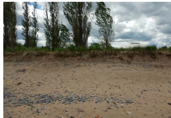
037 - Eroding dune at north end of NMU beach. Location 3.
