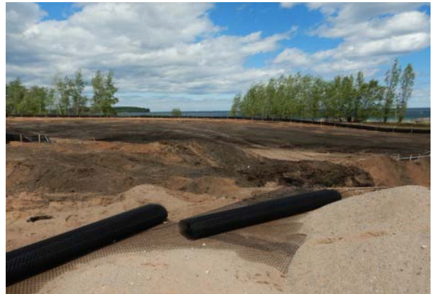
009 - Storm water detention basin being constructed. Location 9.
