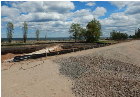
010 - Storm water detention basin being constructed. Location 9.
