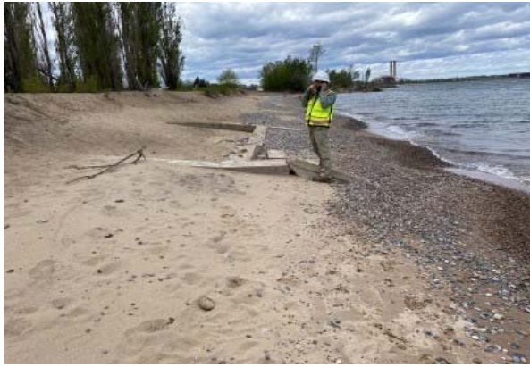
022 - Newly exposed concrete foundation on the NMU beach. Near Location 3.
