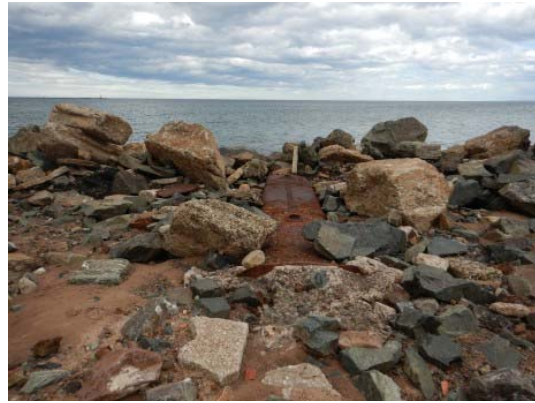
104 - Newly discovered riveted iron box culvert with evidence of tar. Location 11.
