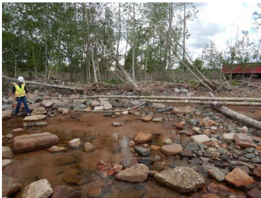
051 - South end of project site, looking south. Location 5.
