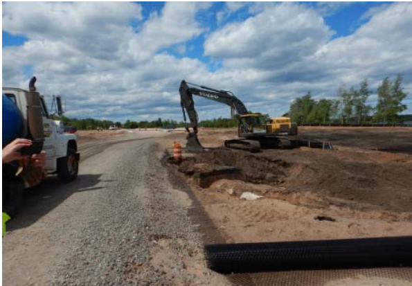
008 - Storm water detention basin being constructed. Location 9.
