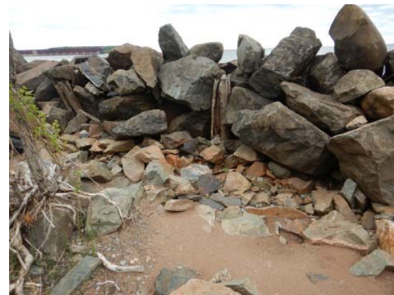
139 - Timber pile in revetment near Location 13.
