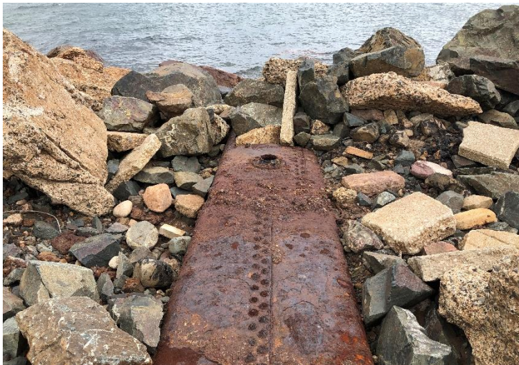
Figure 2.2: Possible Historical Retort Discharge Pipe from Cliffs-Dow Site
