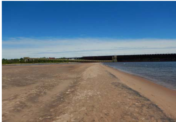
020 - Looking north onto the sand spit at the mouth of the Dead River. Between Locations 19 and 20.
