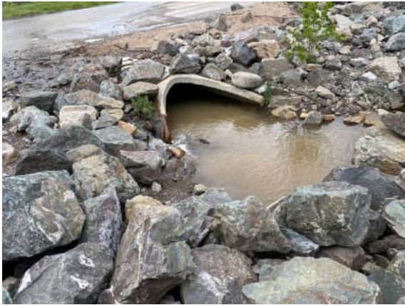
056 - Stormwater outfall at Location 6.
