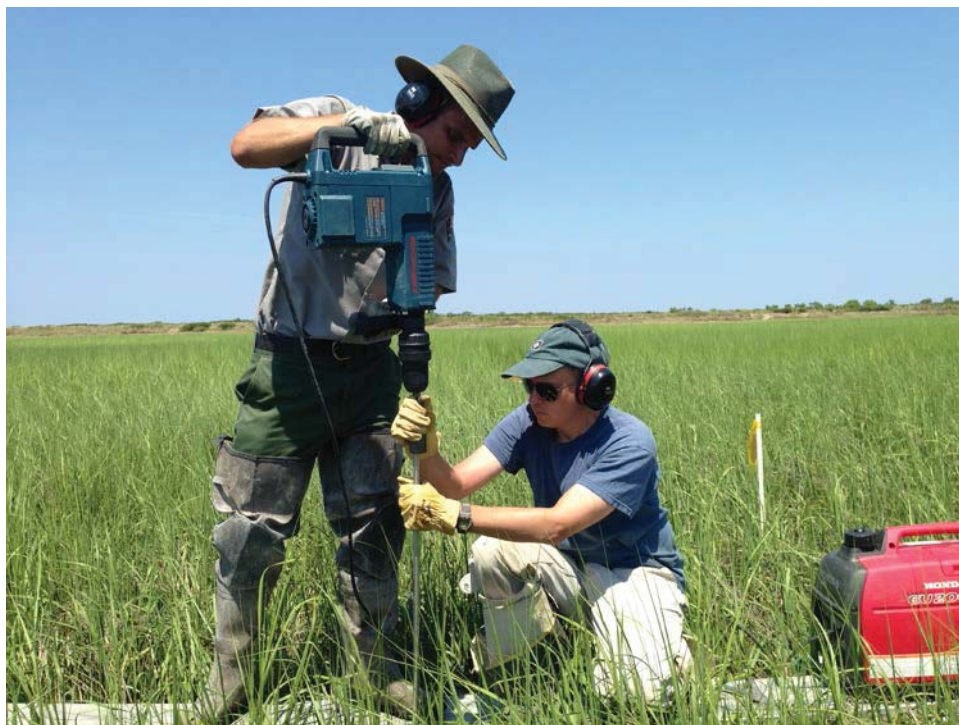
Figure 3.4. Demolition hammer and generator (Cape Cod NS, Massachusetts, USA).
