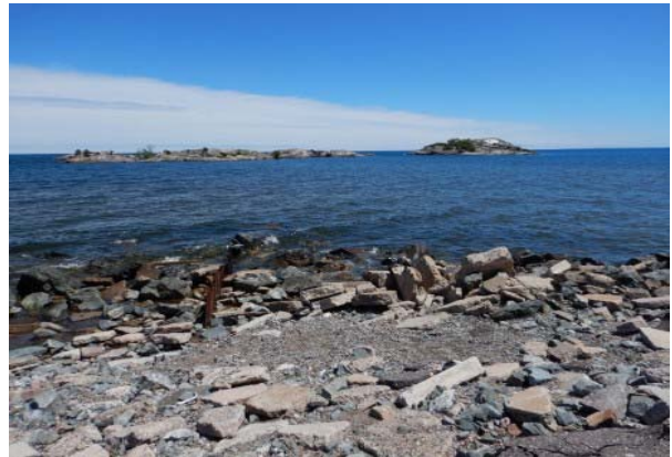
002 - Looking at Picnic Rocks from Shiras Park. Note the remanant SSP groyne on the left. Location 1.
