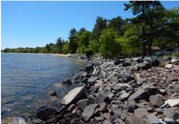
009 - Looking south along the shoreline at Shiras Park. Relatively new armoring indicates ongoing erosion. Location 1.
