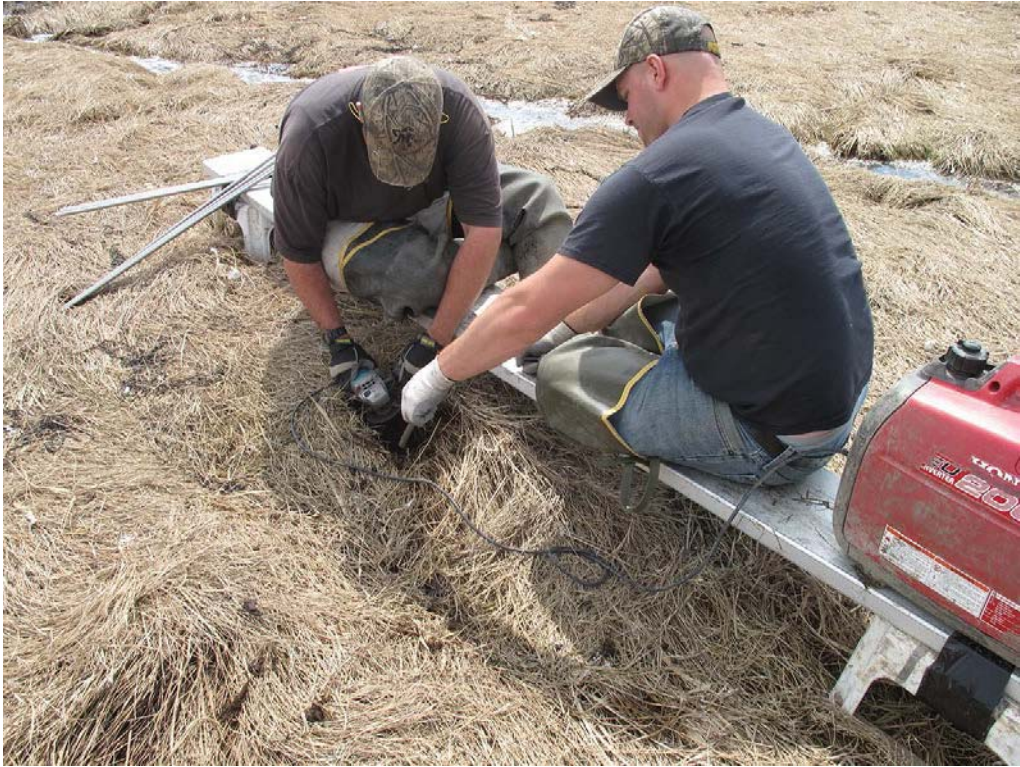
Figure 3.16. Cutting the rod with an angle grinder (Boston Harbor Islands NRA, MA, USA).
