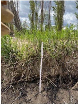
031 - Eroding dune at north end of NMU beach. Scarp is approximately 2' to 2.5' high. Location 3.
