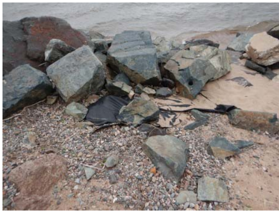
163 - Exposed geotextile. Location 17.
