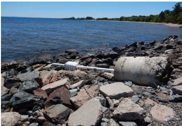
005 - Sign advising swimmers against dangerous currents and water conditions has toppled due to chronic erosion. Location 1.
